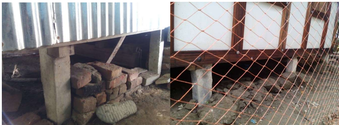
Figure 3. Deep rooted pillar use at the base of the house.
