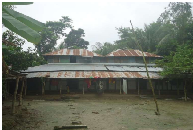
Figure 6. Attached house for increase the strength against cyclone and storm surge.
